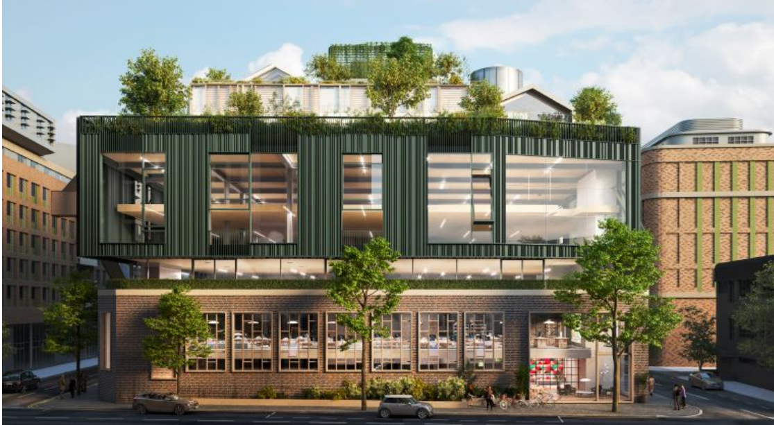
Figure 6 (above): Visualisation of the proposed east façade. A shoulder line is created by the stepped-back nature of levels 04, 05 and 06, while the various pavilions, trees and raised metal drum give the building its eccentric roof profile.
