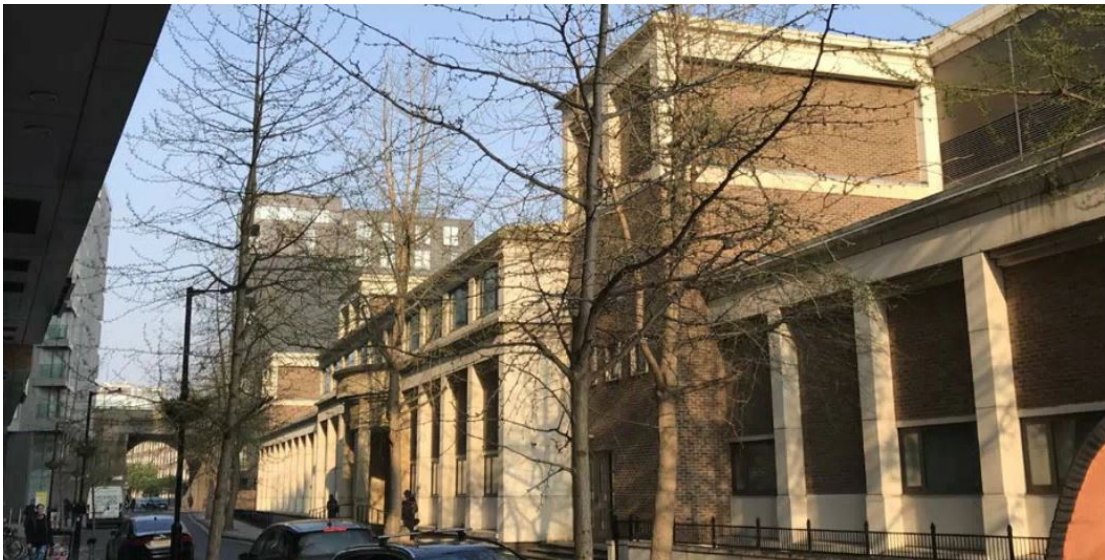
Figure 24 (above): The Pocock Street elevation of the existing Crown Court building.
