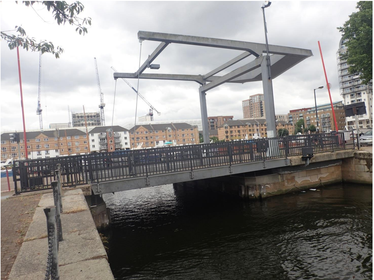
Figure 8 – Rope Street Bridge
