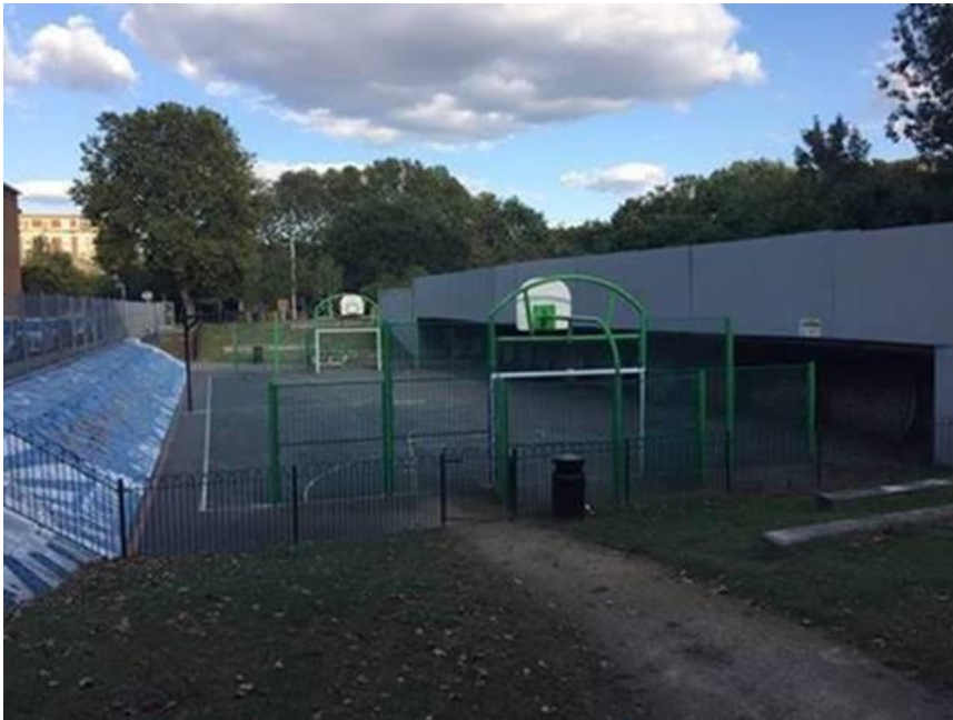
Figure 3: existing pedestrian bridge (right) demolished due to structural issues since August 2022
