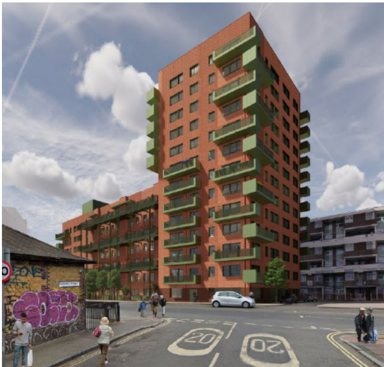
Image: G1 viewed from junction of Hornshay Street and Ilderton Road
