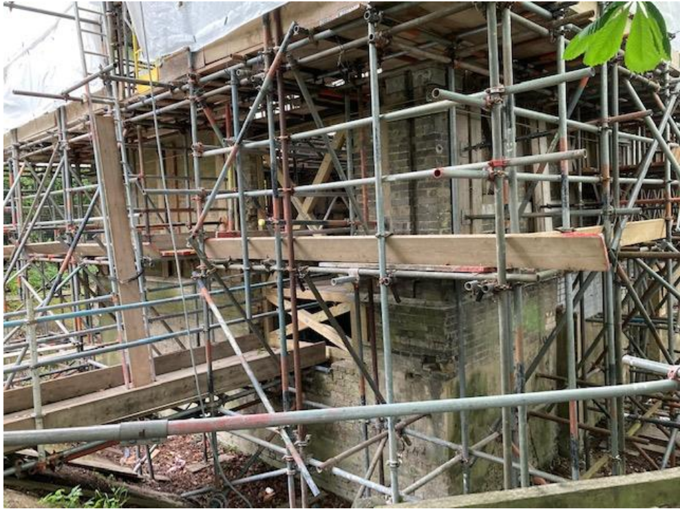
Above: scaffold with concrete weighting supporting the building
