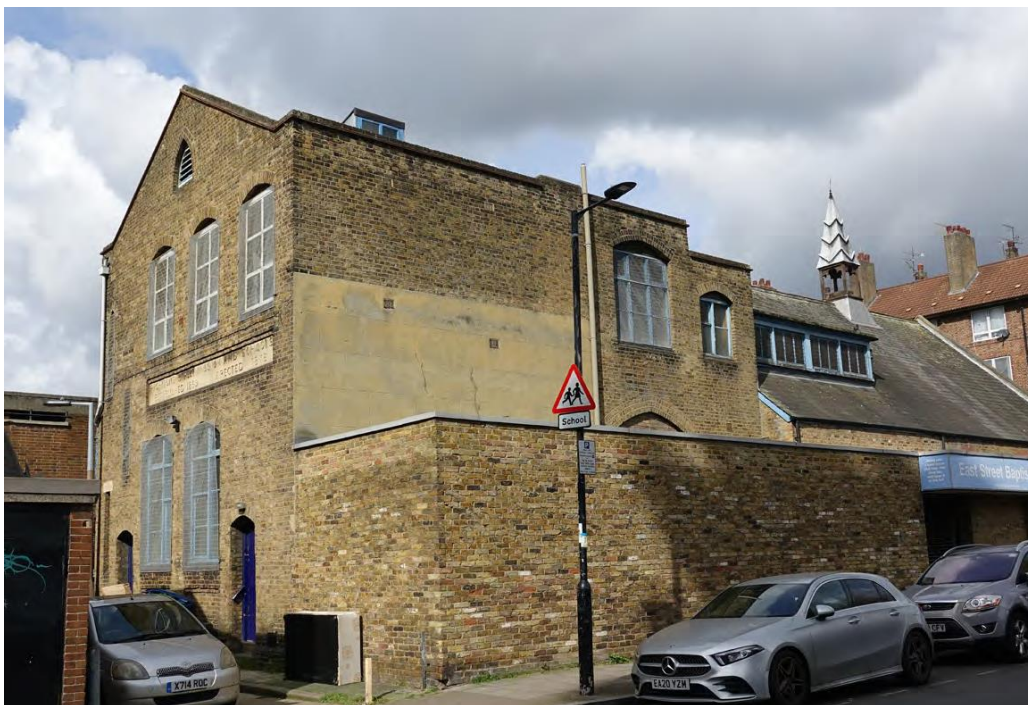
View of the Ragged School (1875) with the 1974 extension of the church in the foreground.
