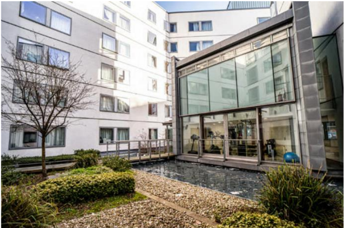
Image – existing courtyard
