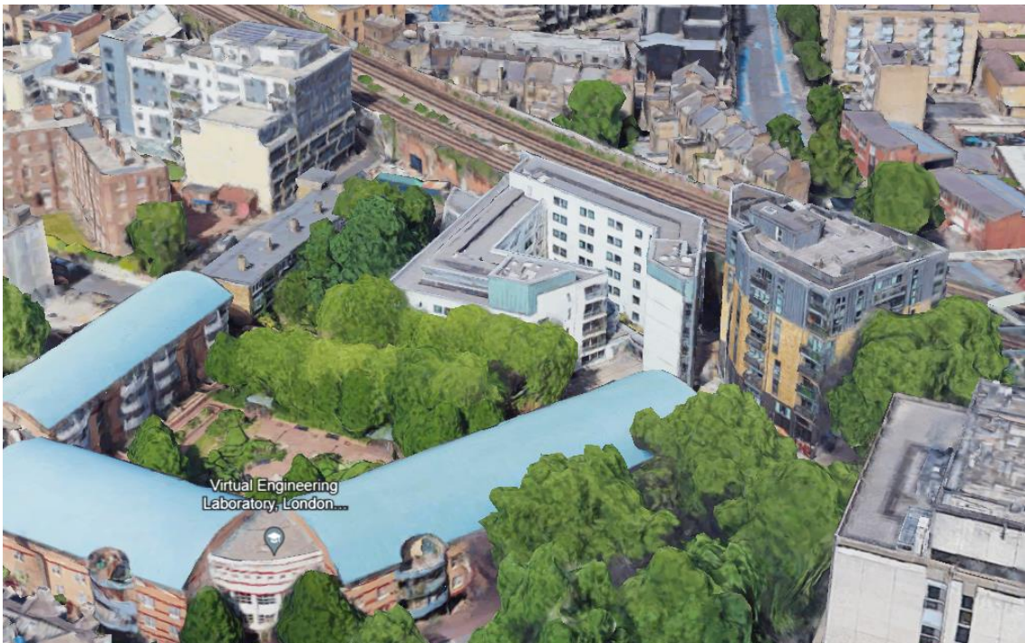
Image – aerial view from the south
