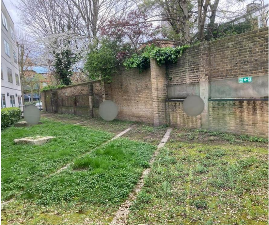
Image - wall to existing rear / north boundary
