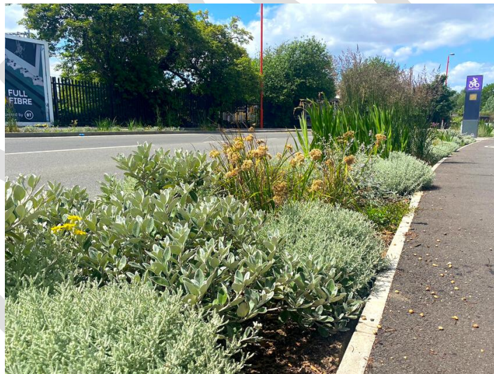
Forest Road, Meristem Design, Rain Gardens/ SuDS
