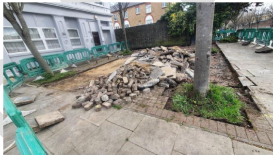
De-paving for the Octopus Garden, Dunton and Lynton Roads, 2022
