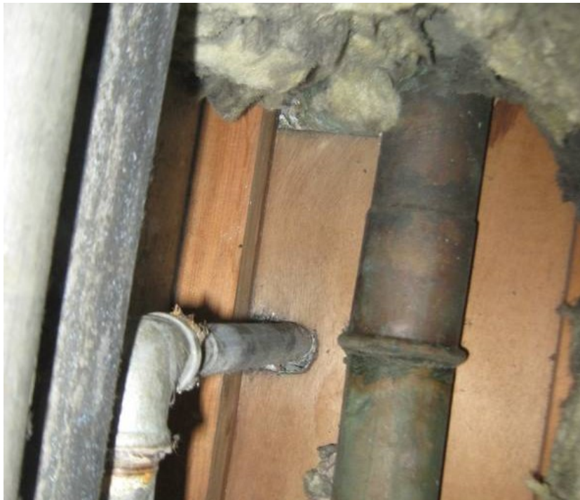
Photo 14 - Lower level duct – plywood panel.
