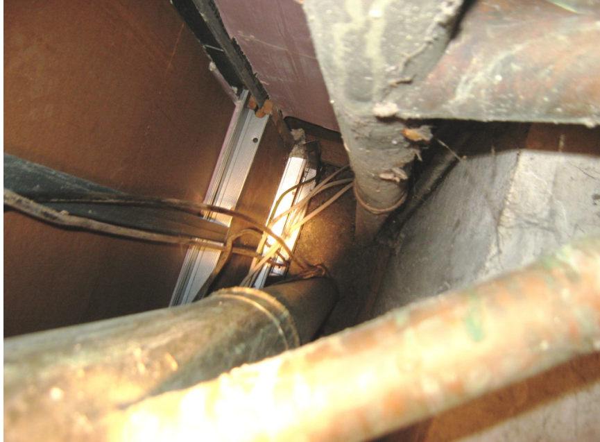
Photo 6 - Partition to adjoining property (bathroom services duct).
