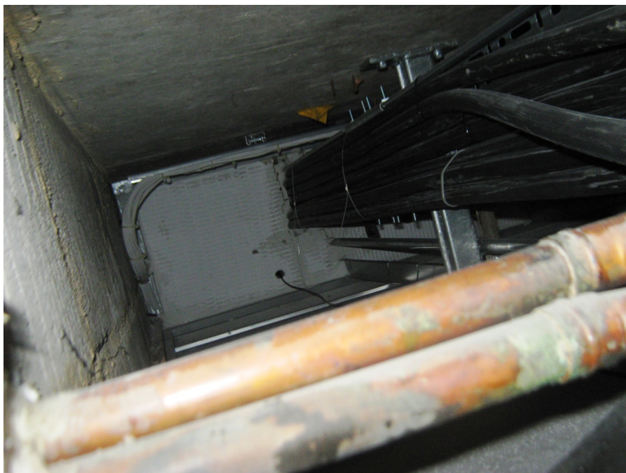
Photo 1 - void above suspended ceiling
