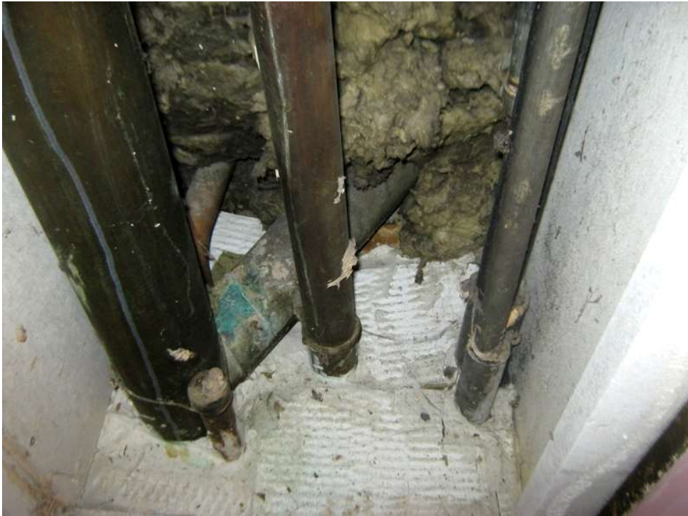
Photo 12 - Lower level duct exposed. Intumescent pads to concrete floor slab.
