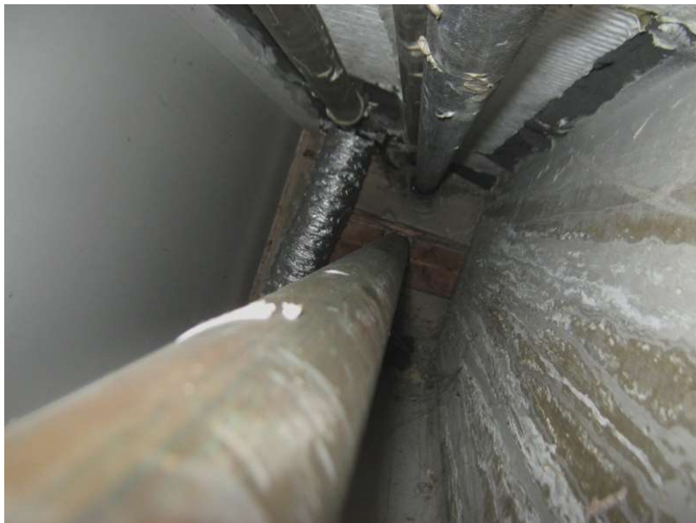
Photo 10 - Top of upper level duct.
