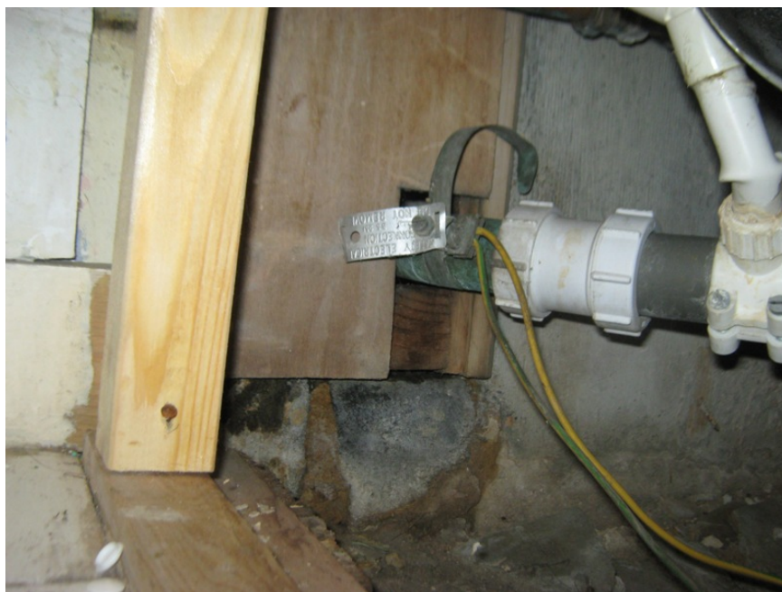
Photo 5 - Plywood panel behind bath.
