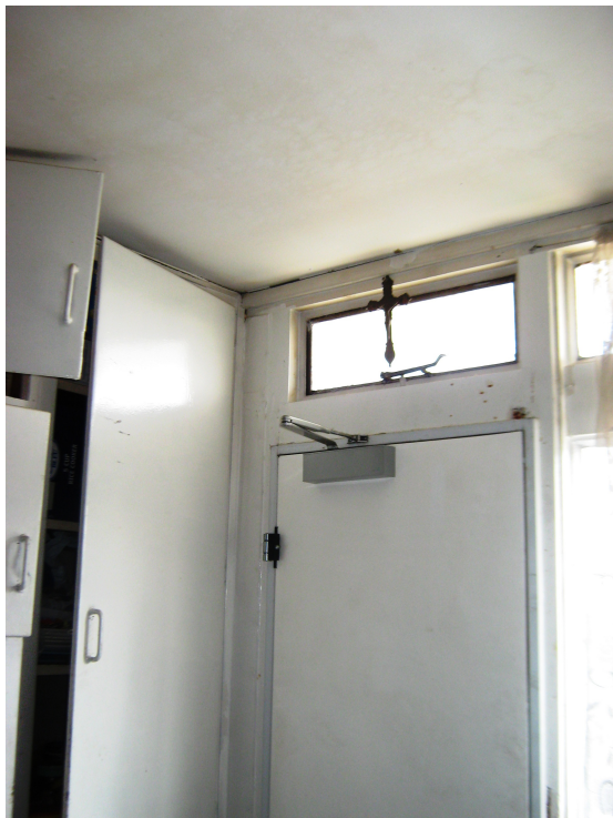
Photo 15 – Plywood panel (behind escape Cupboard).
