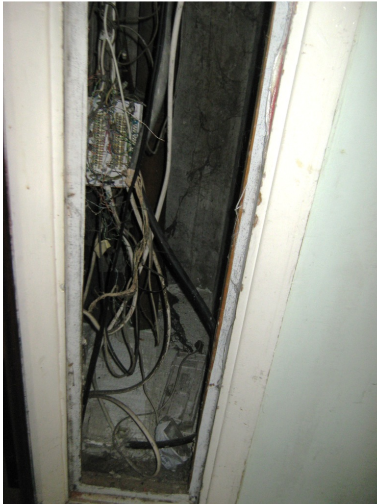
Photo 2 - Common area redundant riser duct - Fire-stopping
