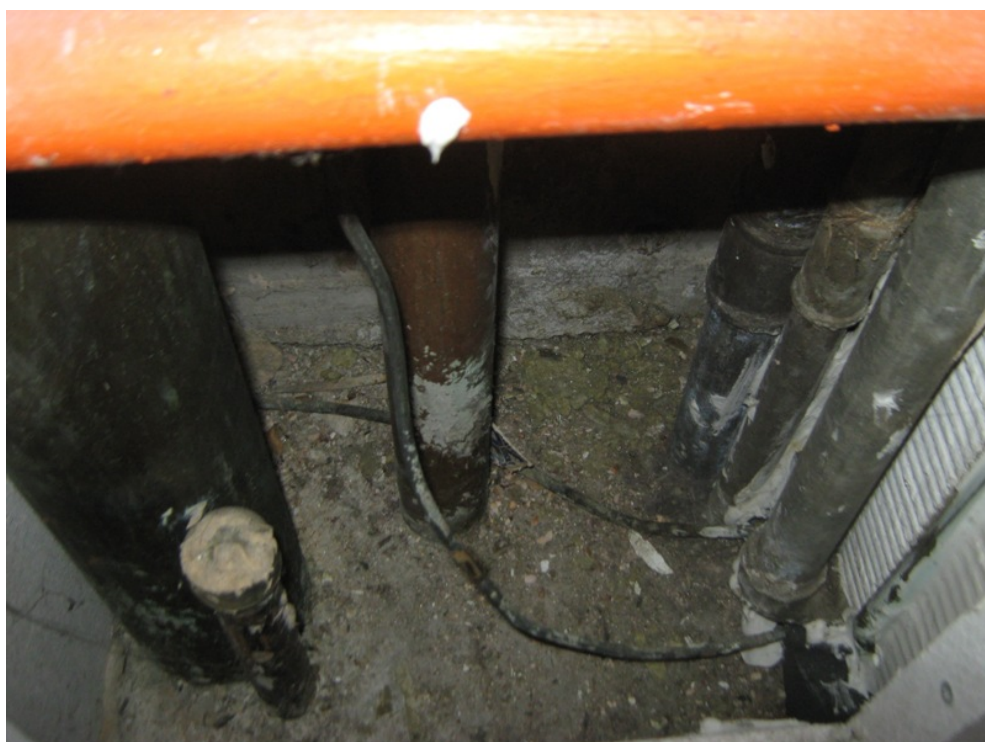
Photo 11 - bottom of upper level duct.
