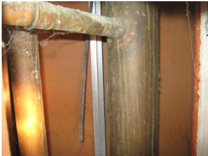
Photo 7 - Inside bathroom duct, showing partition.
