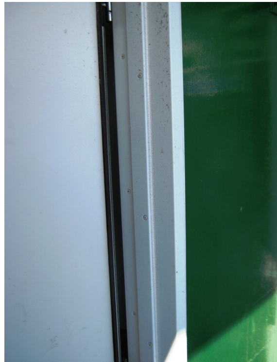
Photo 16 – Plywood panel on external emergency escape balcony.
