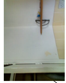
Insulating board as partition wall
