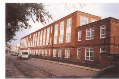
Figure 2 – 1926 addition to the school, fronting Grove Lane
