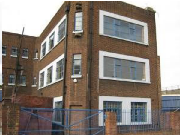
After remedial works
