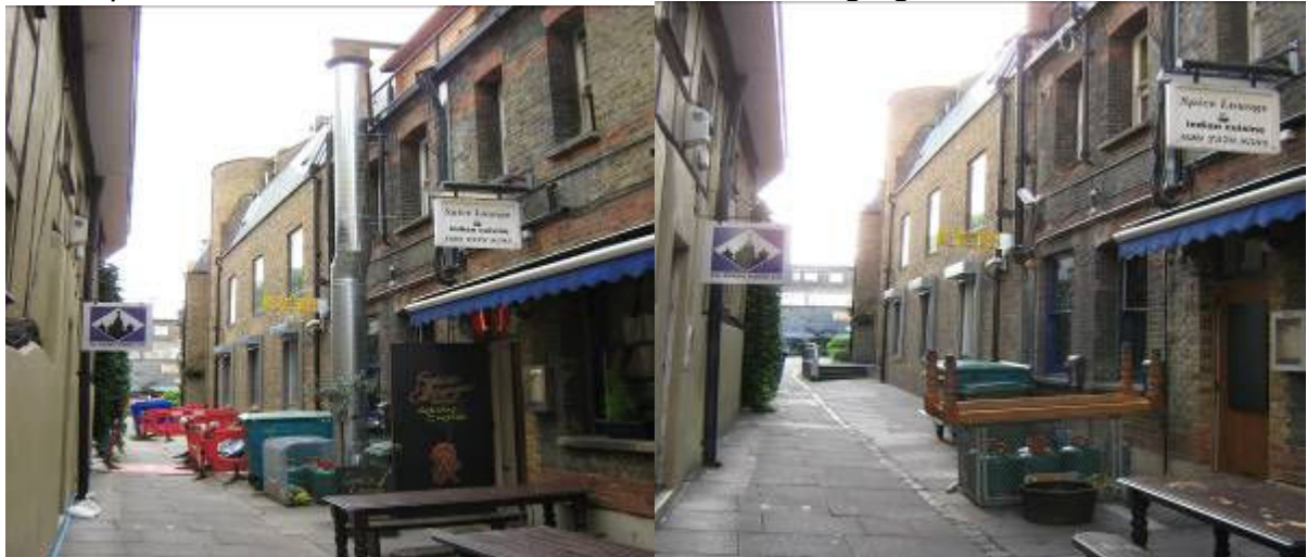
Unauthorised extraction duct affecting street scene
