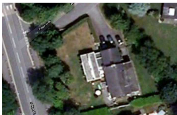
Photo-1: Aerial image showing grassed area before it was converted to gravel under PD rights
